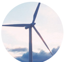
Wind power generation
